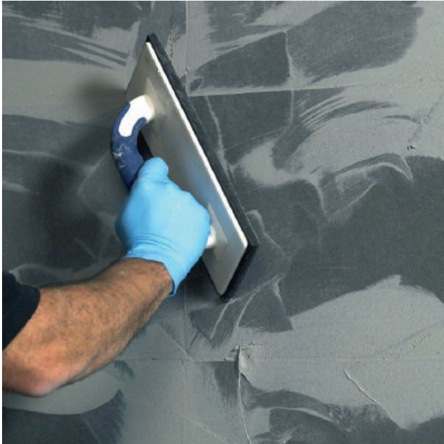
Workable grouting within approx. 40 minutes.
